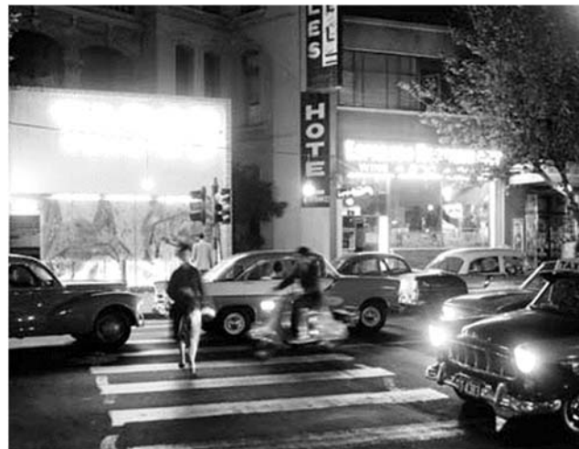
Figure 19: Night-time photograph of Darlinghurst Road in front of No 24 Darlinghurst Road, 1961. With neon lights Greyeagles Hotel is proclaimed as “Tabou” while the late 1950s addition by Frank Kolos is shown as a restaurant serving wine well into the night, indicating the cosmopolitan nature of Kings Cross. Image: NAA_A1200 L38208
